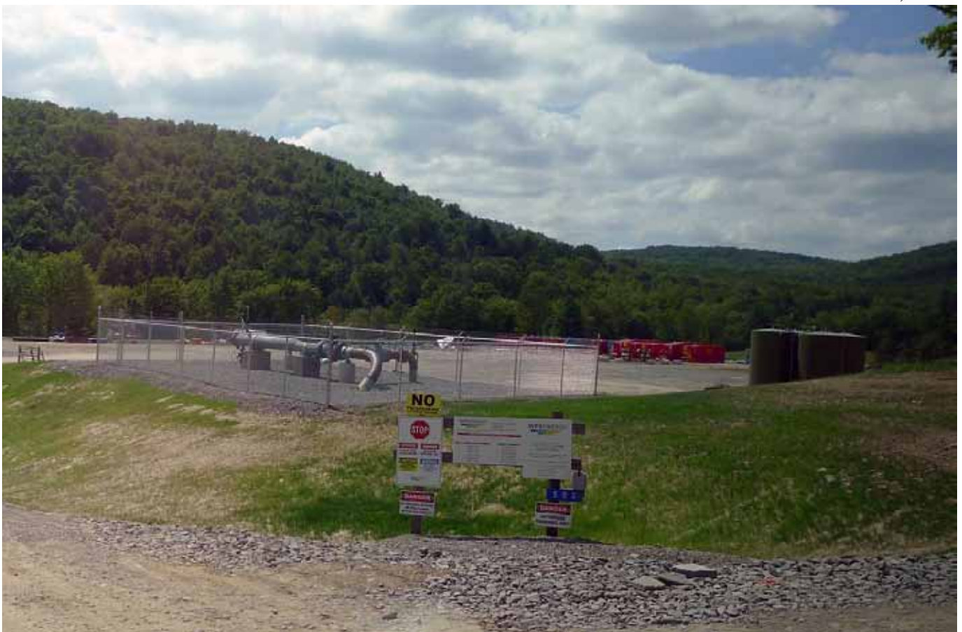
A fracking well site in Franklin Township near Montrose and Dimock.
