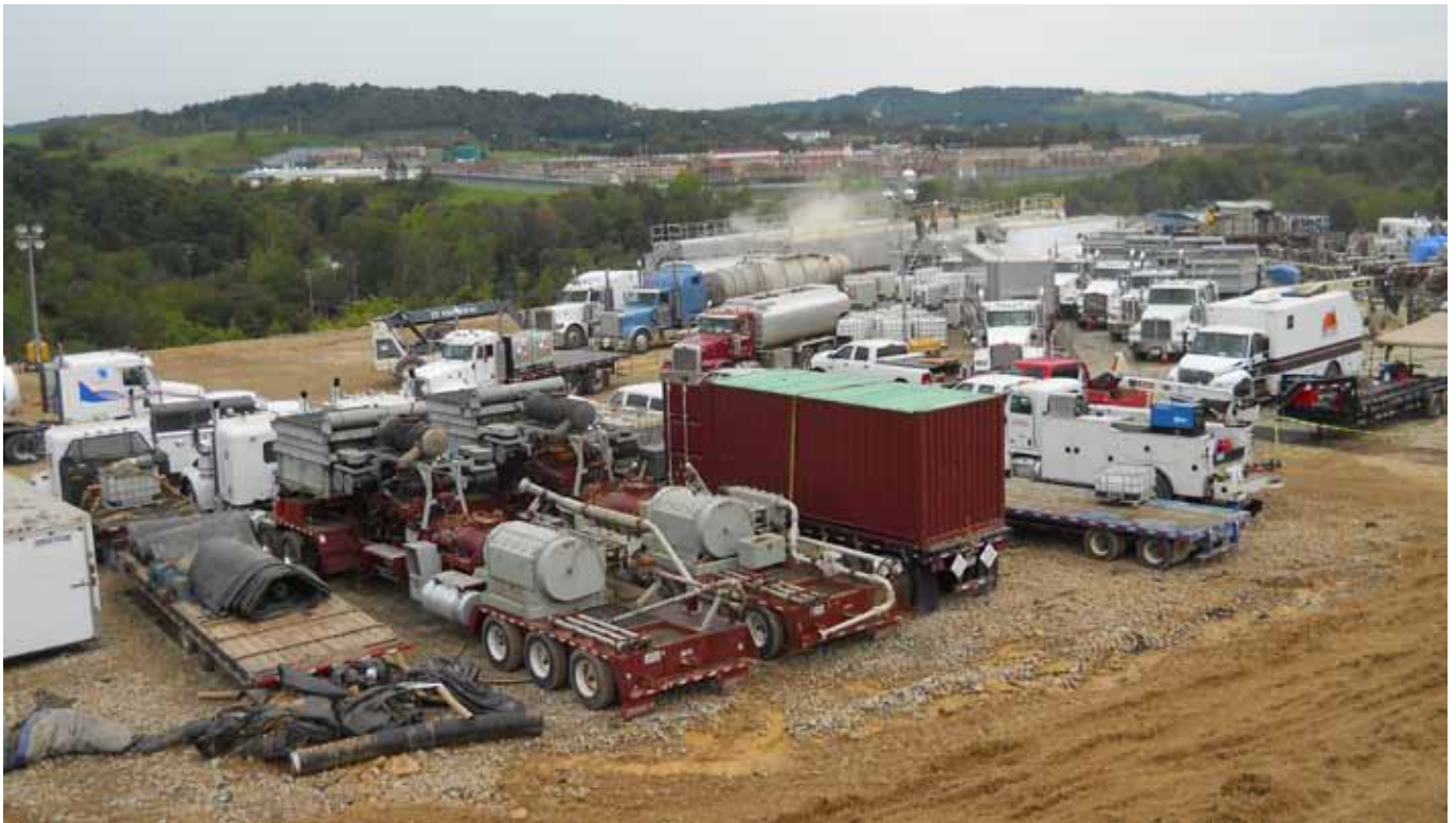
A drill pad in southwestern Pennsylvania during fracking operations.
